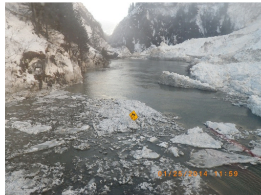
Fig. 1: Damalanche. Avalanche dammed lake flooding Richardson Highway.
