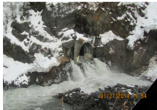
Fig. 5: Old highway tunnel allowing drainage
